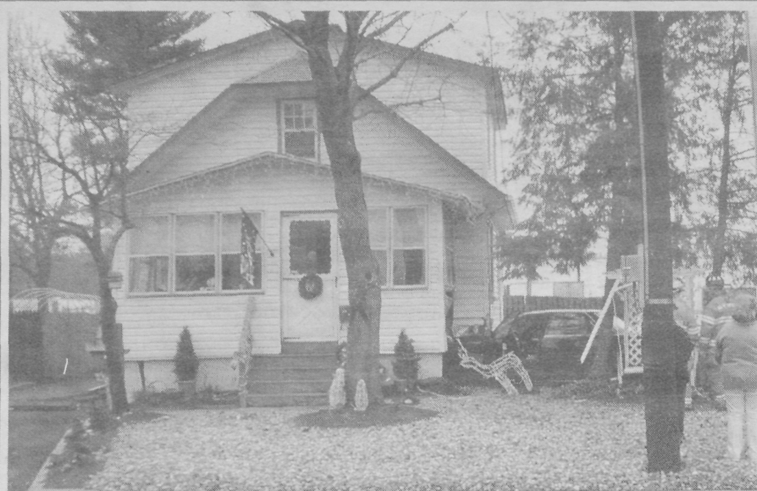
An accident on Tuesday morning left this home damaged after a vehicle traveling eastbound on Oak Tree Avenue struck the median divider and a tree at Halls Warehouse, then continued on crashing into the enclosed front porch of the house causing major structural damage. The home was unoccupied at the time of the crash. The car was driven by Patricia Torres, 35, of Plainfield. Neither she nor her passenger, Jacqueline Mendoza, were injured. Torres was charged with being an unlicensed driver and careless driving.
