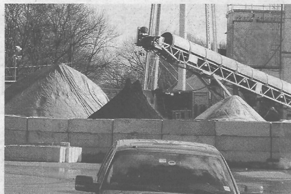
Soil is discharged from a conveyor belt after being treated in the Low Temperature Thermal Desorption Unit at the Cornell-Dubilier Electronics superfund site.
