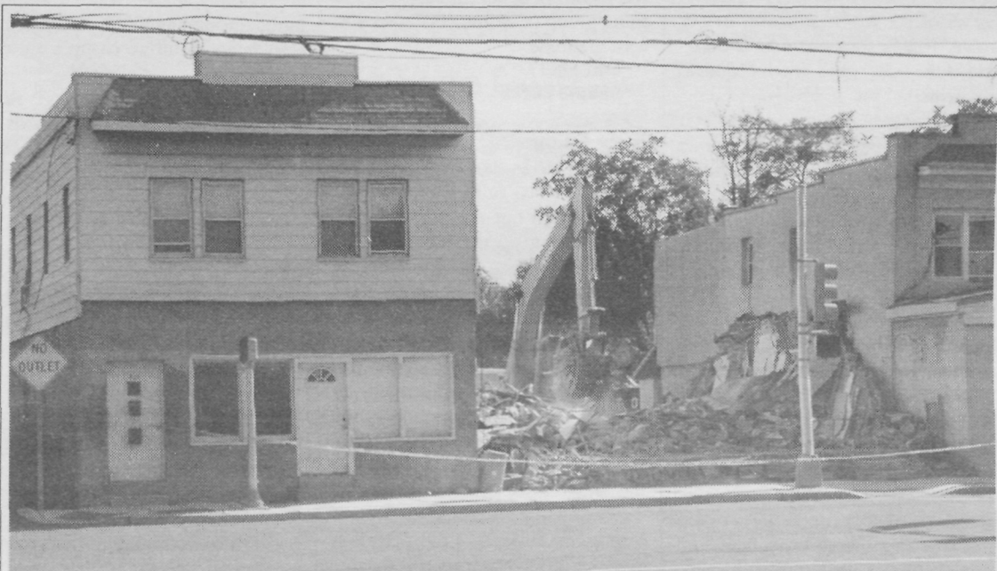
Re-structuring of the intersection at New Market Avenue and Hamilton Boulevard continues with the demolition of the first of three buildings on Hamilton Boulevard. When completed, the new route will allow trucks to cross Hamilton Boulevard to Spicer Avenue without making two sharp turns.
