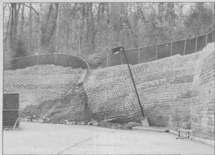
Flood waters resulted in the closing of the Clinton Avenue Extension (above left). Above right, the collapse of the retaining wall behind Sears Hardware on Oak Tree Road will close Woodland Avenue for at least two weeks.
