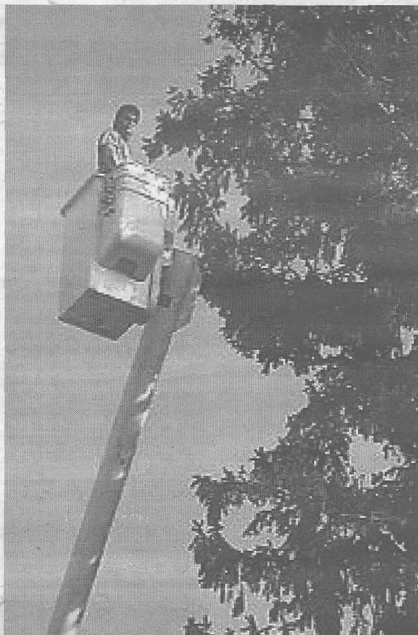
McCriksen brought in a crane to prepare its tree for the lighting ceremonies on Dec. 12. The tree is 79 feet high, has over 13,000 lights and burns over 10,000 watts of electricity. Feeding the lights are nine circuits at the base of the tree that go up the trunk into five enclosed junctions.
